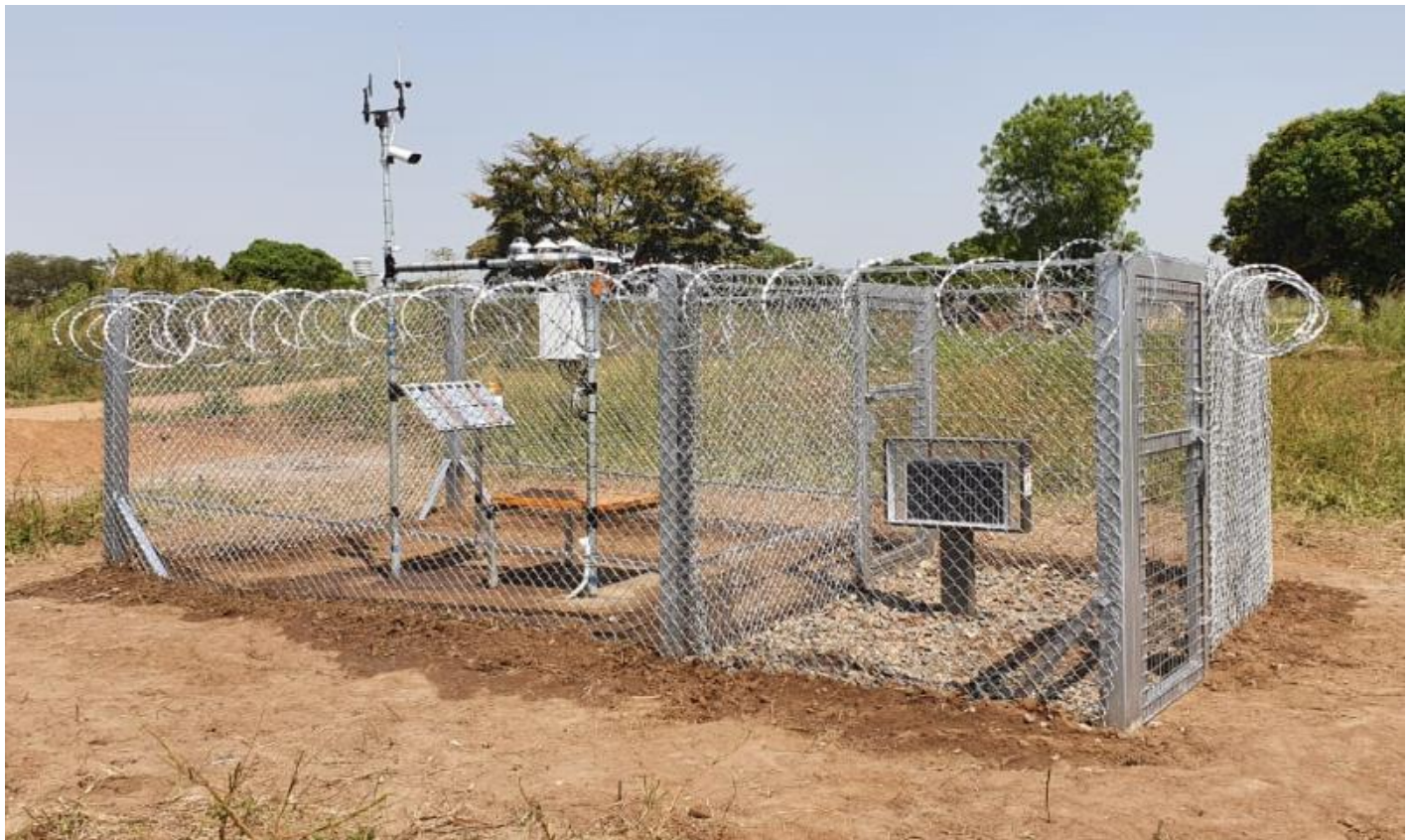
Figure 1: Wadelai on-site solar and meteorological measurement station
