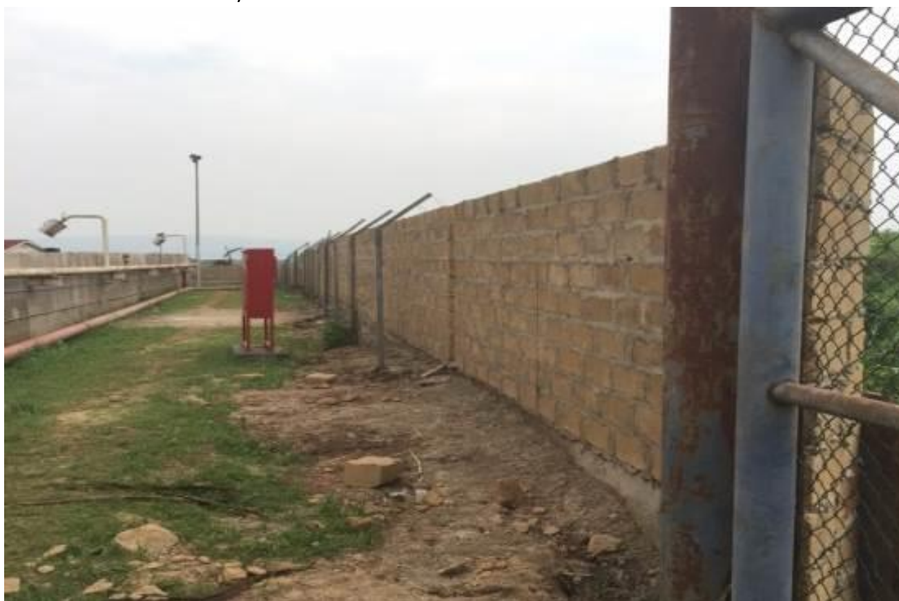
Fig. 32: Fence at JST under Construction
