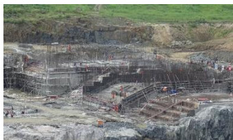
Fig. 15: Spillways partially concreted to elevation 1026 and 1029 ft respectively (September 2015)
