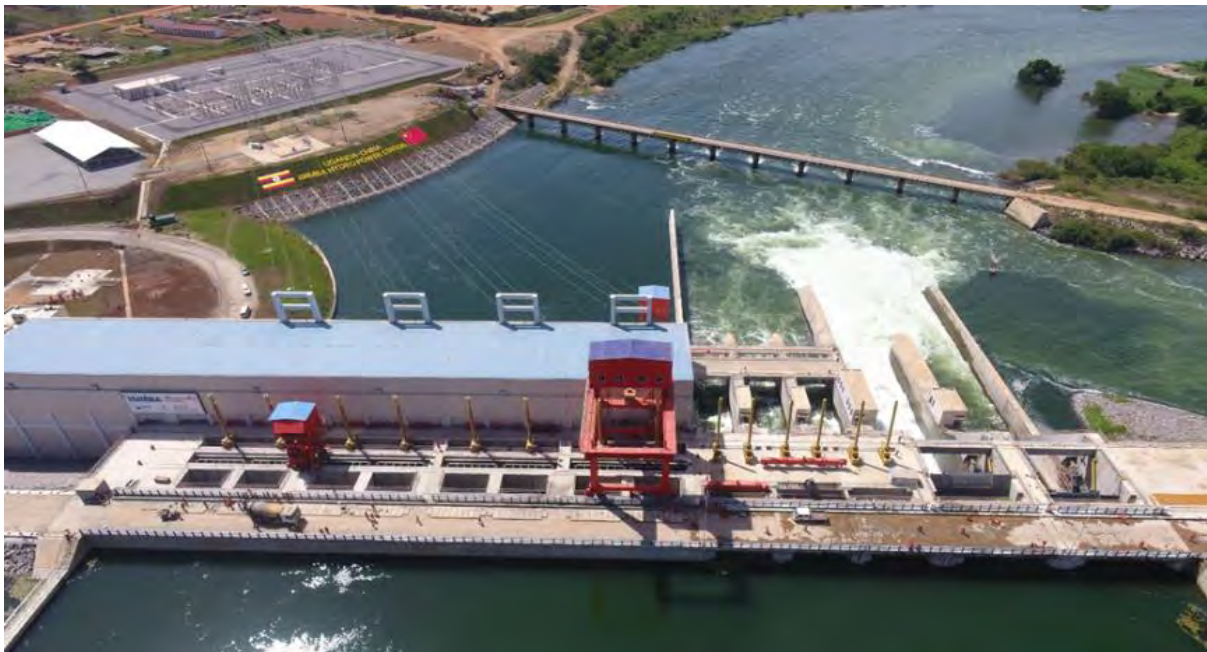
Picture 3: An Aerial view of 183MW Isimba Hydropower Plant
